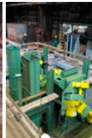
Komore s turbinami
